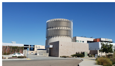
Facilities and Central Plant
